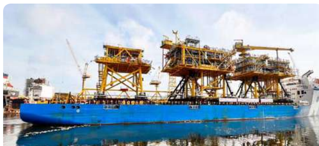
Tyra West modules and bridges delivery
