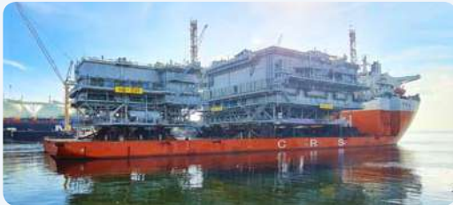
Hornsea 2 Offshore Wind Farm substations
