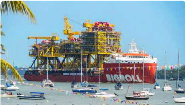
Sailaway of the Tyra East modules and bridges
