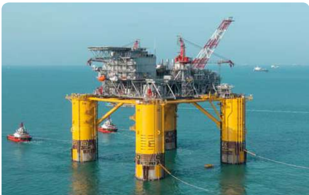
Successful delivery of the Vito RPF – the first of two newbuild FPUs – in December 2021
