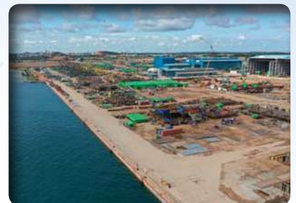
SEBMCORP MARINE BATAM YARD (PT. SMOE INDONESIA)
