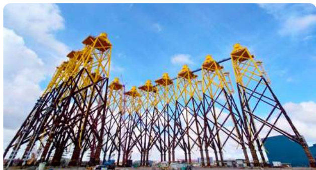
Fabrication of 15 wind turbine jacket foundations for the Formosa 2 Offshore Wind Farm
