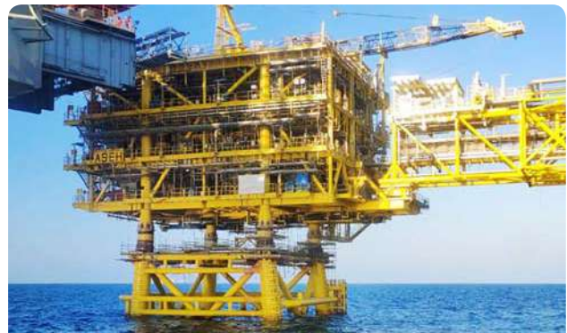
Offshore works in progress on two wellhead platforms and bridges for the Gallaf Batch 2 Project at the Al-Shaheen Field
