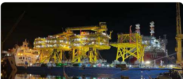
Delivered final phase of the Tyra Redevelopment Project with the completion of two wellhead topsides, one riser topside and two bridges for the Tyra West Field in 2022
