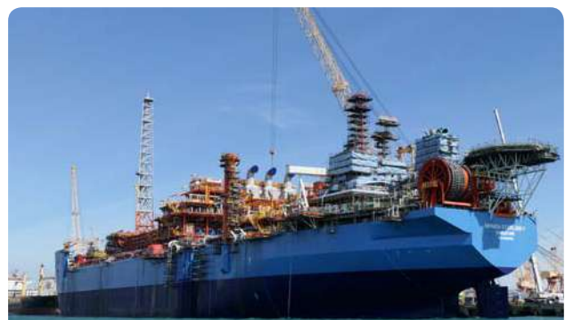
Armada Sterling V FPSO conversion
