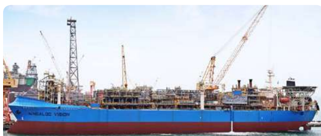
Performed FPSO upgrading for Ningaloo Vision
